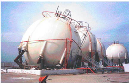
Collapsed spherical tank due to corrosion
