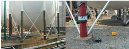
FOCUS+ used to measure corrosion of tank legs
